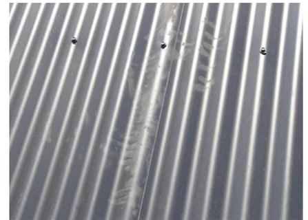
**Figure 2. Roofing with sunscreen damage**
